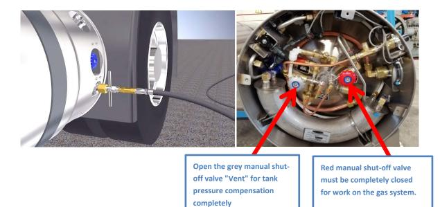
Figure 6-5: Blow-off device and manual shut-off valves; source: ZDK
